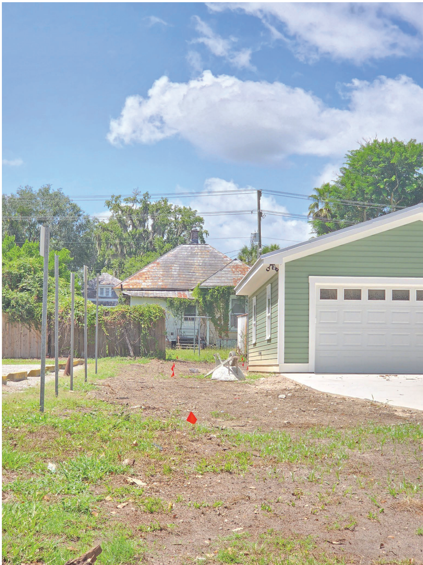
The eastern property line of the property where a section of the fence will be installed facing south
