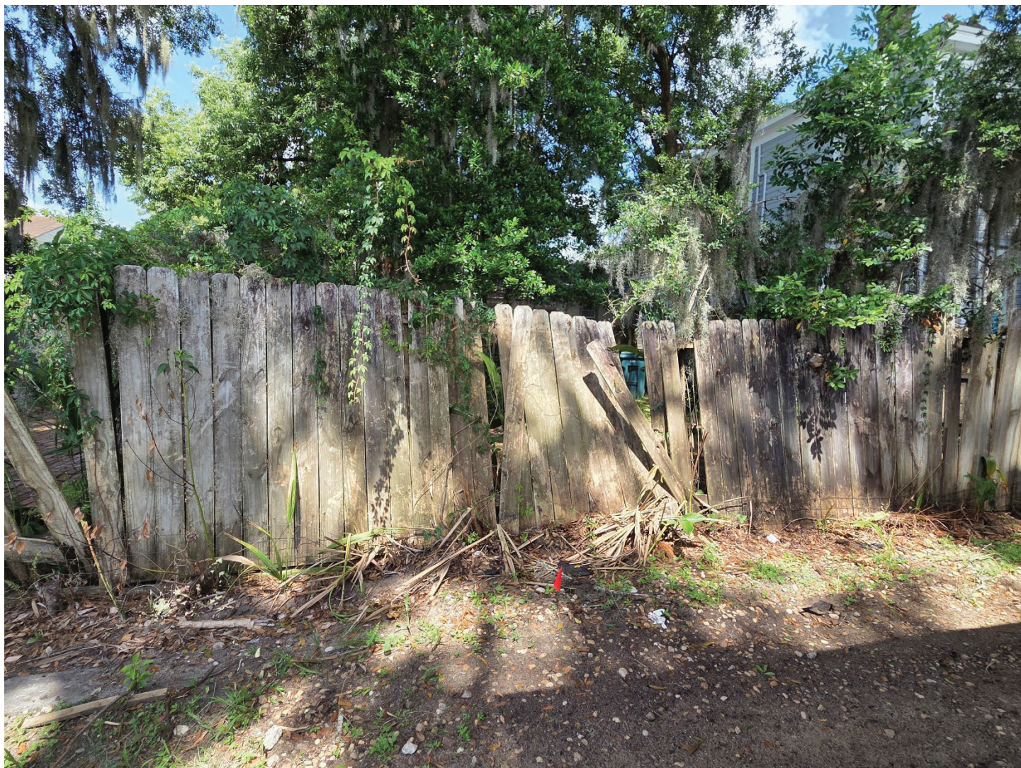
The fence along the western property line
