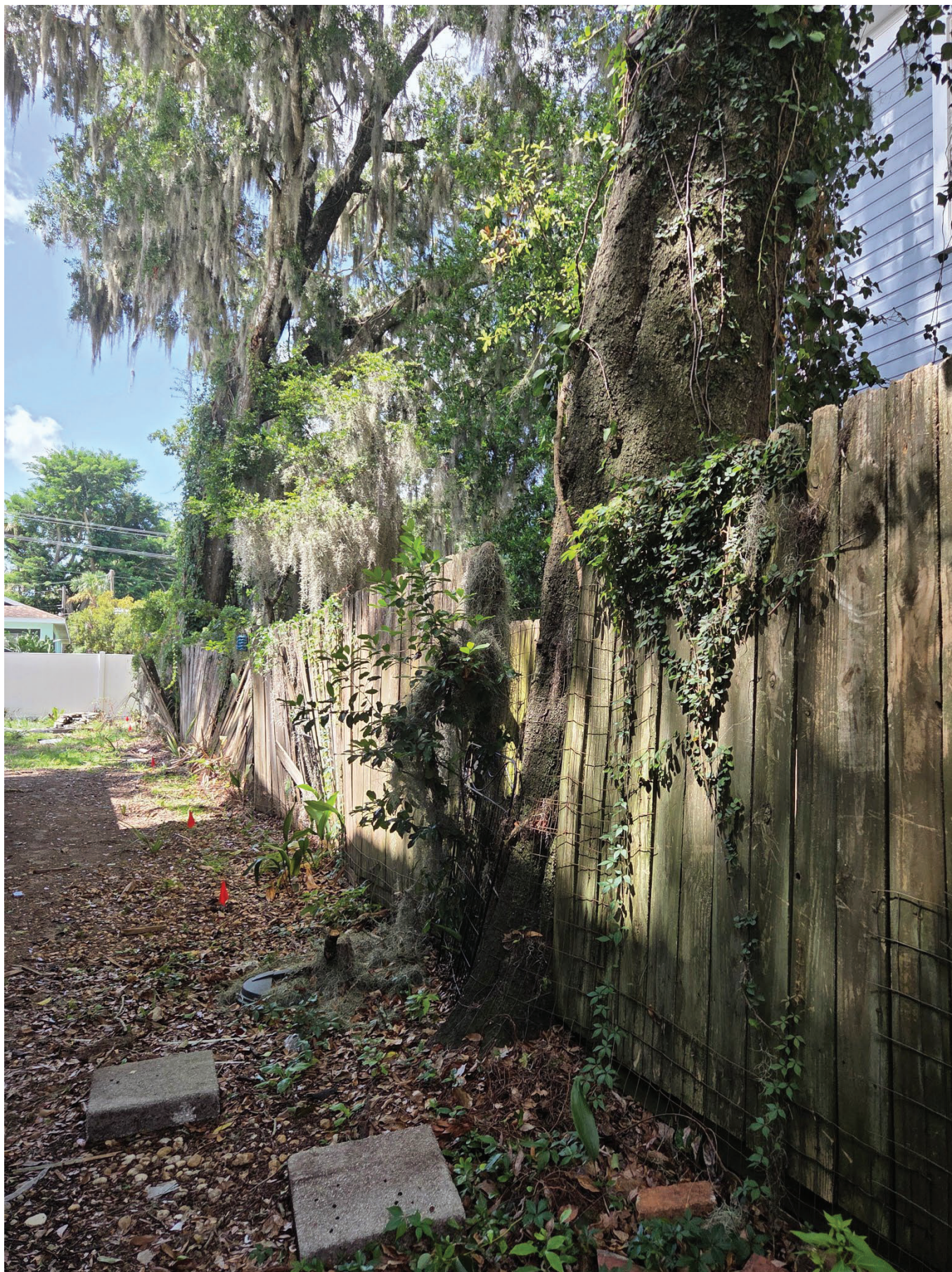
The fence along the western property line
