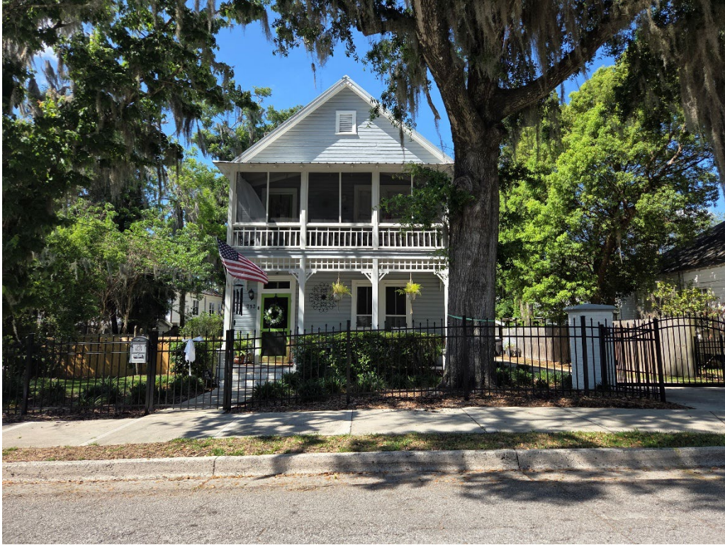
Subject property (facing north) from SE Second St.
