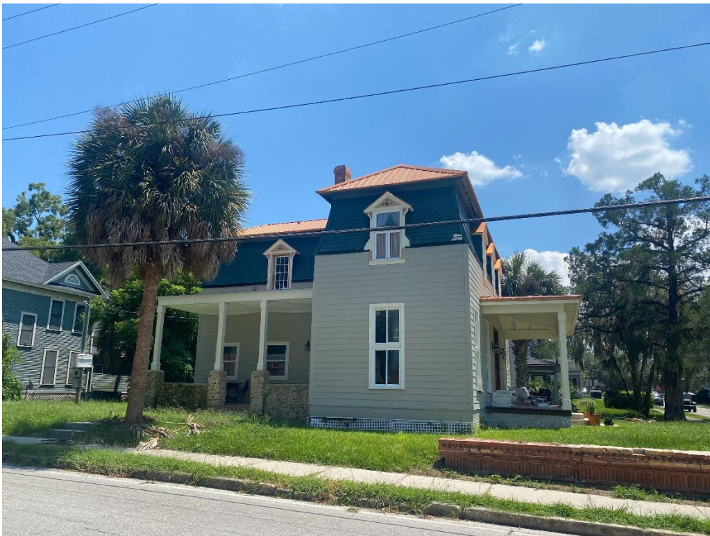
Facing south onto the subject property on
