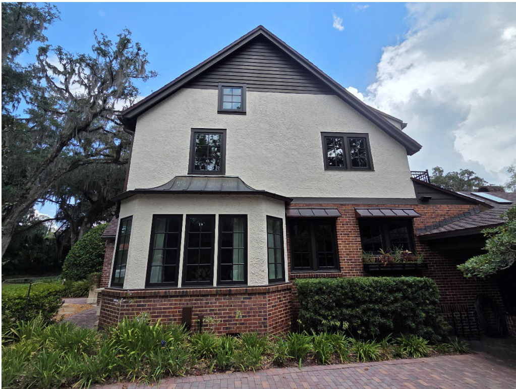
The three windows that will have awnings installed above three windows with similar awnings
