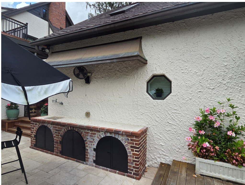
Other areas on the property with similar copper awnings
