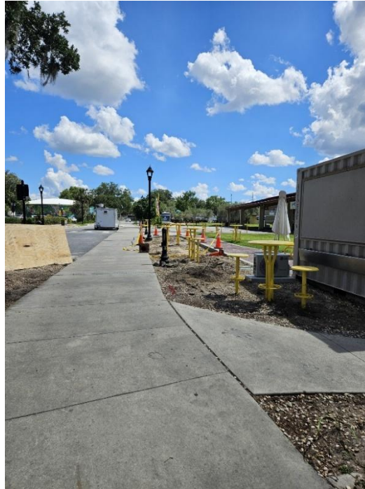
DOWNTOWN MARKET - IMPROVEMENTS IN-PROGRESS
