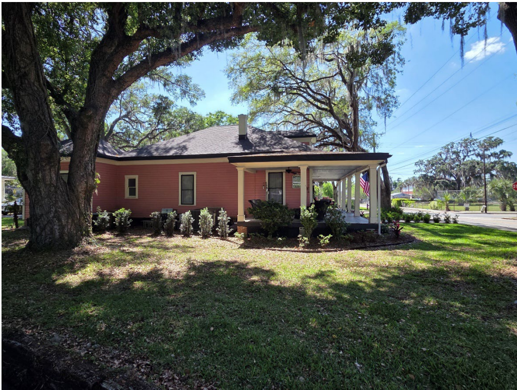
Subject property (facing west)
