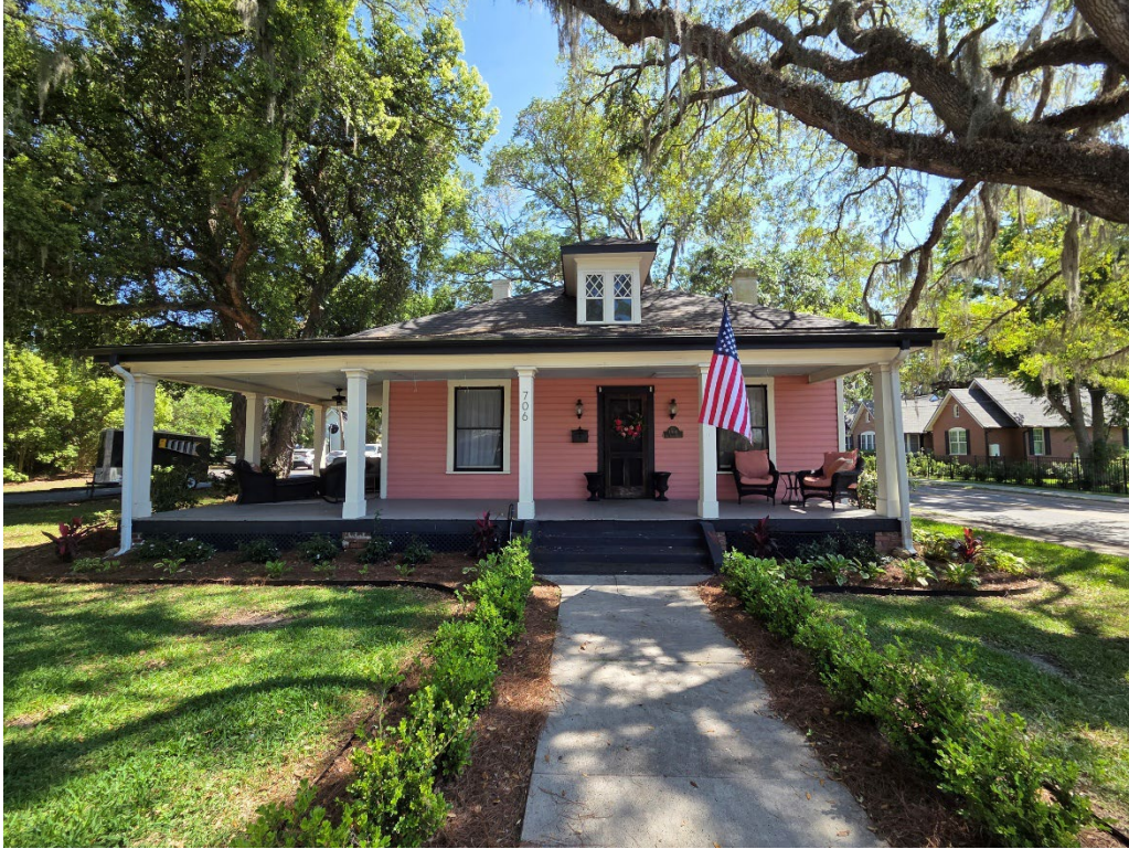
Subject property (facing south) from SE Fourth St.
