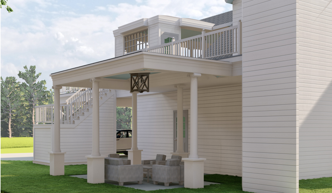
Ground-Level Pergola: Constructed over existing concrete pad. Columns replicate existing architectural rhythm and proportions. Roof and materials match main structure.
