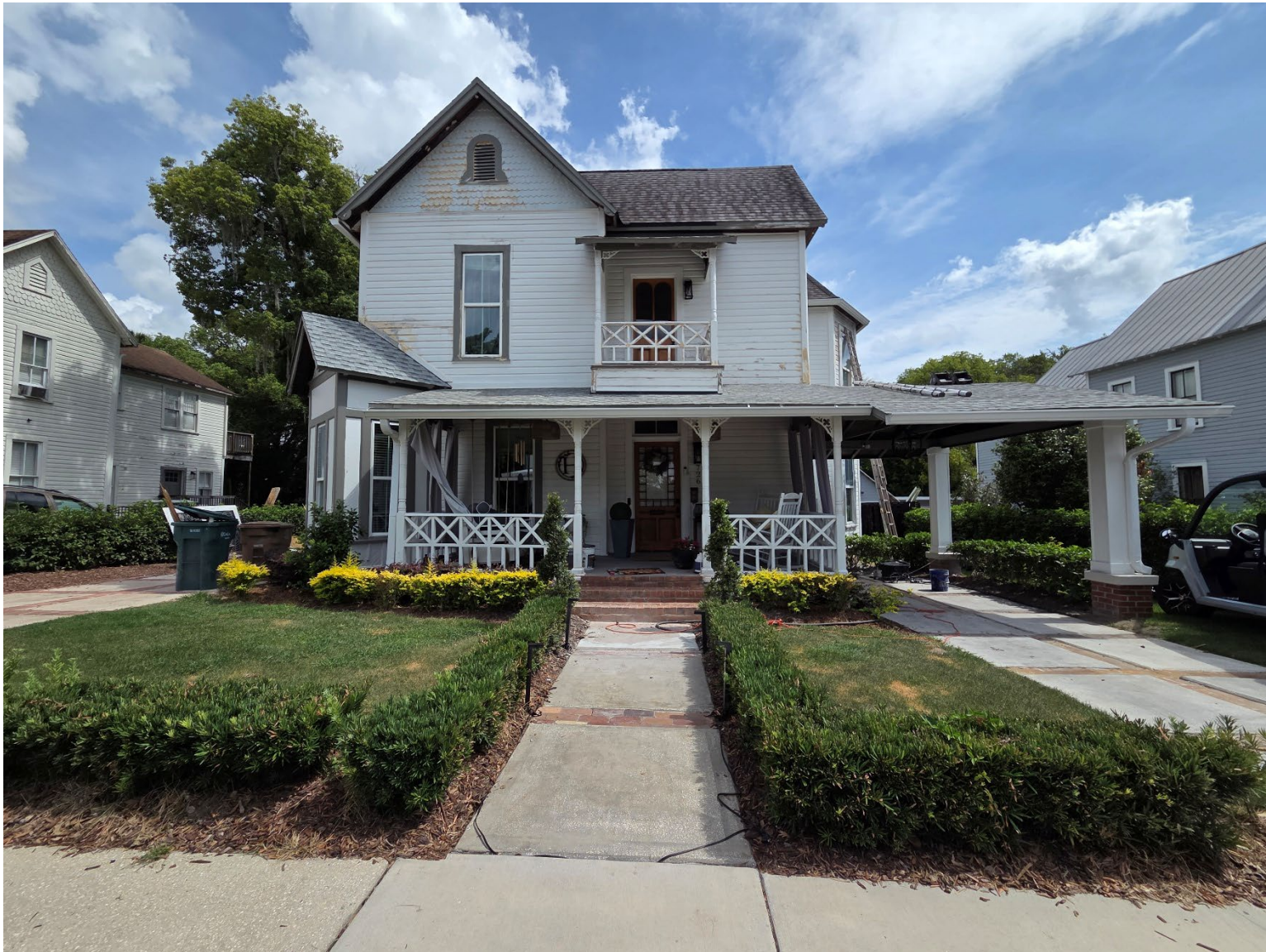
Photo 1: SE 726 SE 3rd Street from SE 3d Street facing south
