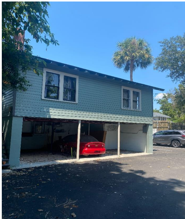
In the rear yard of 709 E Fort King Street, facing north viewing the existing accessory structure.
