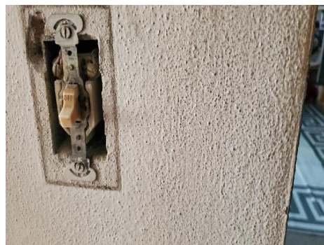
923-5 Plaster Typical Interior Walls/Ceilings
