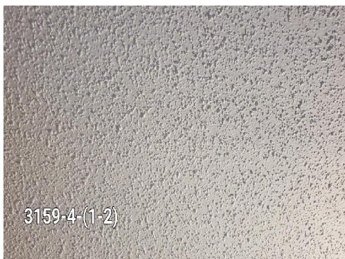
3159-4 Ceiling Surfacing Texture/Cream (2% Chrysotile) Typical Interior Ceilings
