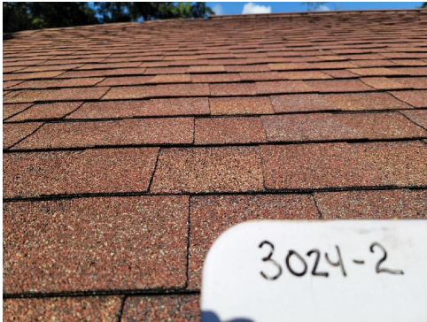
3024-2 Asphalt Shingle Typical Exterior Roof
