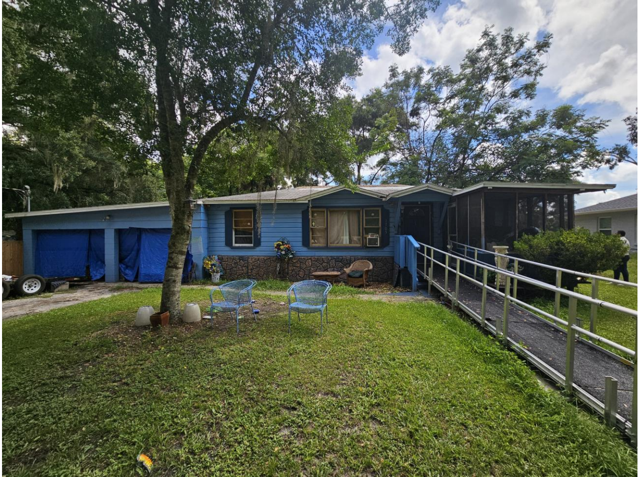
Image 1-View showing the existing conditions at the front of the property.
