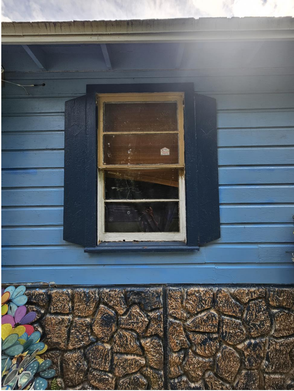
Image 3- View of existing window.
