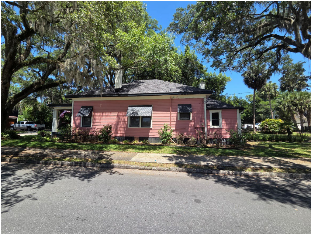
Subject property (facing east)
