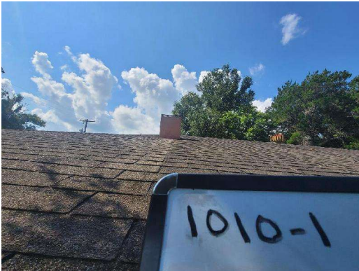
1010-1 Asphalt Shingle/Tar Typical Exterior Roof
