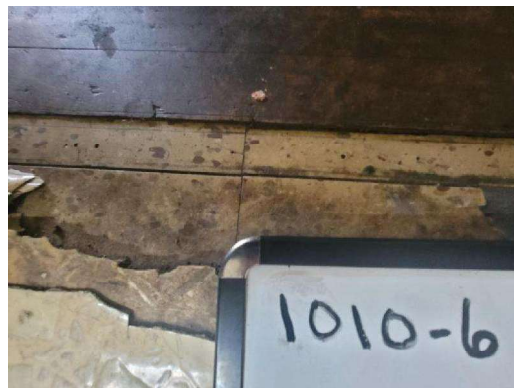
1010-6 12"x12" Floor Tile/Tan (2% Chrysotile) Mastic/Black (3% Chrysotile) Interior Kitchen/Bottom Layer (Appx 190 sq ft)
