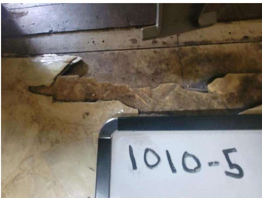
1010-5 Rolled Flooring/Beige (10% Chrysotile) Adhesive Interior Kitchen/Middle Layer (Appx 190 sq ft)
