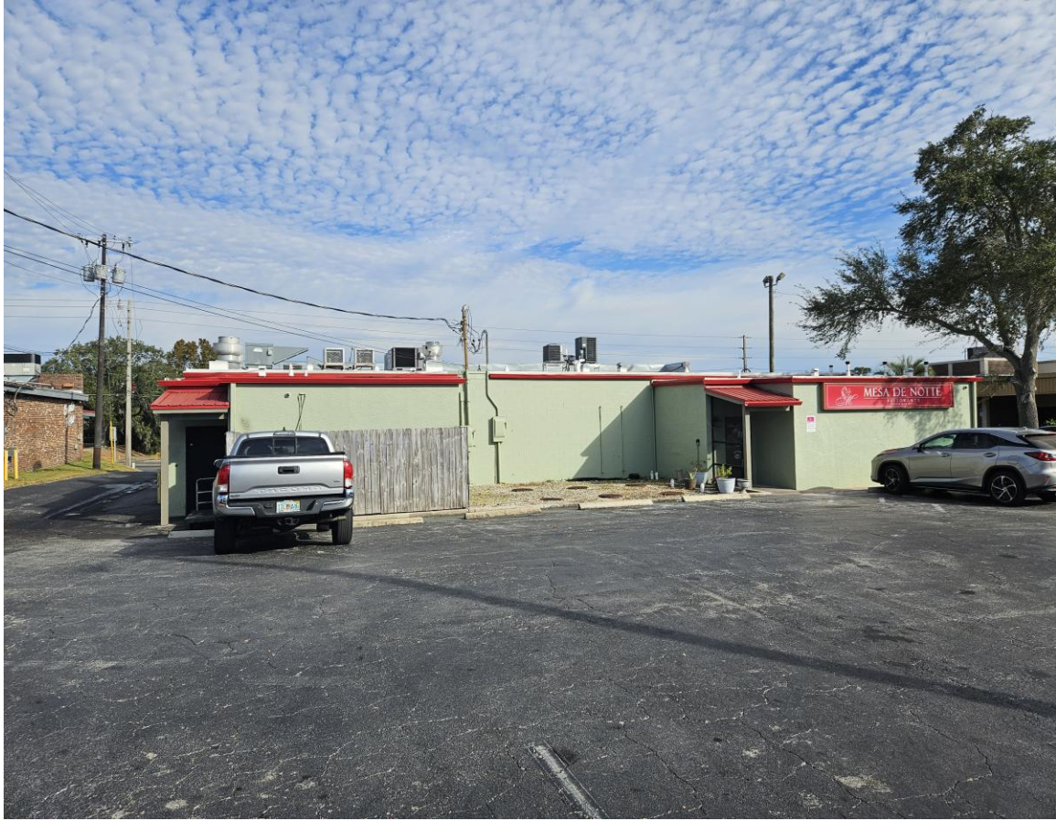
Image 6 – Existing condition of parking lot
