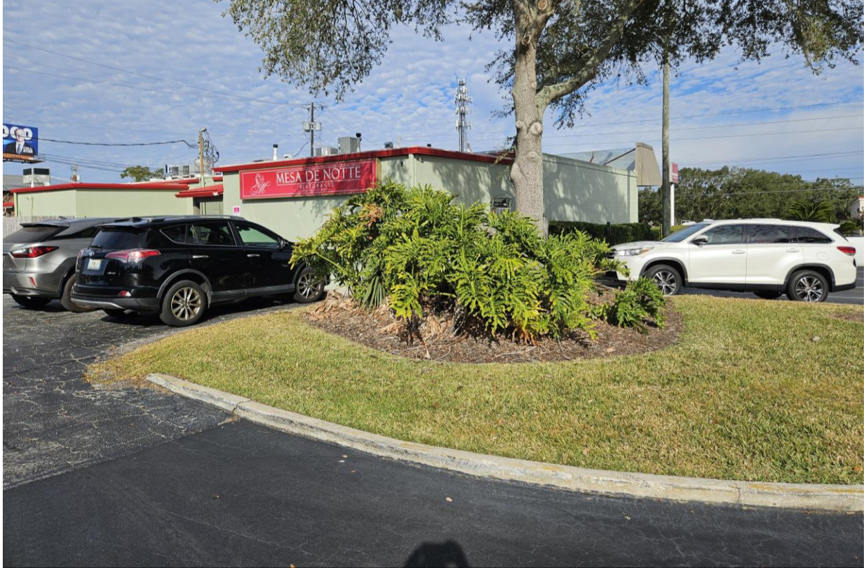
Image 3 – Existing condition – Rear entrance
