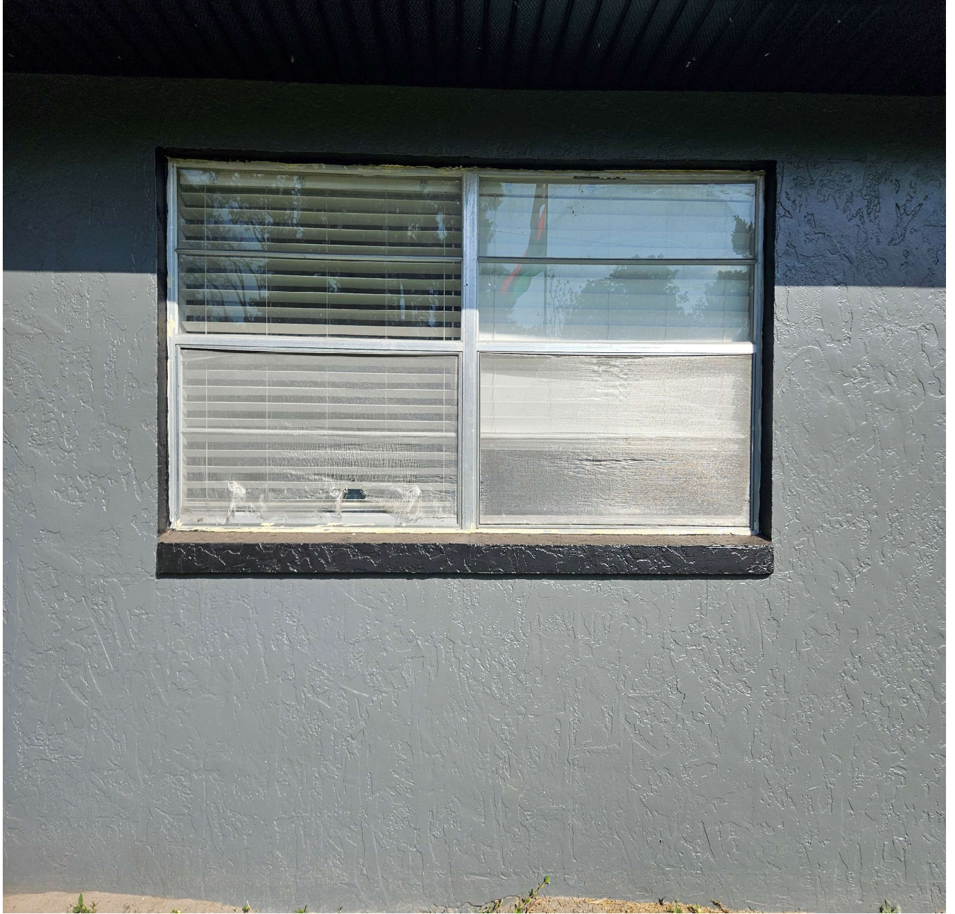
Image 2- View of existing window.
