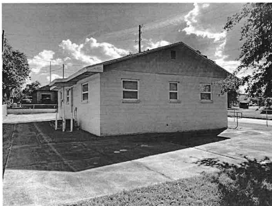
Additional view of Building 3 - Youth/Health . This photo shows the typical construction features (painted block with gable composition shingle roof). View is to the southwest.
