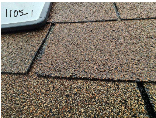
1105-1 Asphalt Shingle/Tar Typical Exterior Roof
