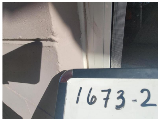
1673-2 Caulk Typical Exterior Windows
