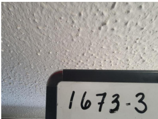
1673-3 Popcorn Texture Interior Bathroom Ceiling
