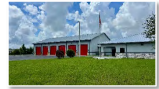
EMS Central Station Marion County BOCC
