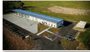
SS Shores W.W.T.F. Maintenance Building
