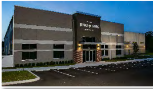
Jing Tang Herbal Office & Warehouse
