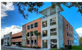
Parking Garage City of Ocala
