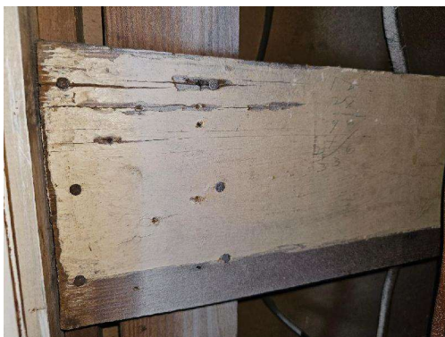
Hallway(005) A-Wall, Left Wood Closet Shelf Support Lead-Positive, Deteriorated
