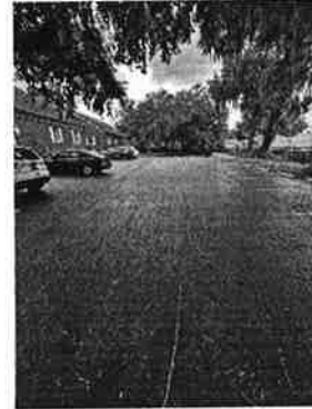
Rear Parking Lot
