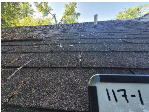
117-1 Asphalt Shingle/Tar Typical Exterior Roof
