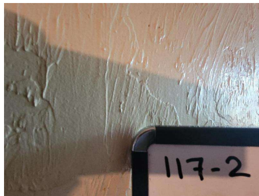
117-2 Drywall/Joint Compound Typical Interior Walls/Ceilings
