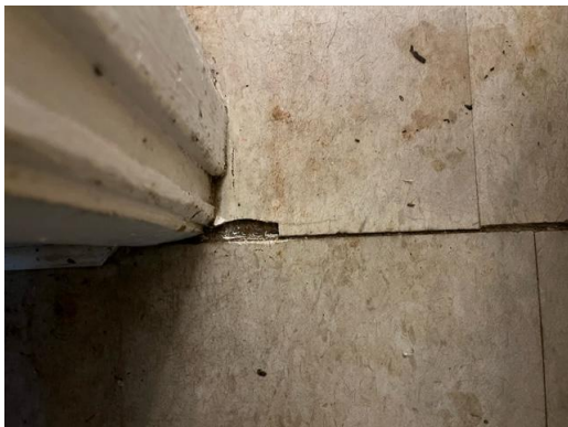
2013-1 12"x12" Floor Tile Mastic/Black (2% Chrysotile) Typical Interior (Approx 1000 sq ft)
