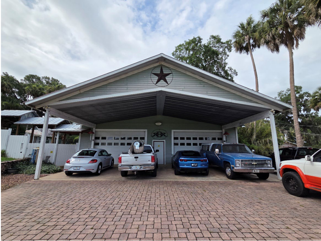
Subject property (garage) from NE 3 rd Street facing south
