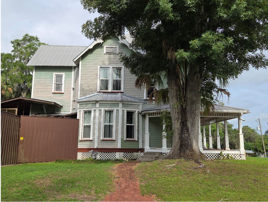
Subject property facing west
