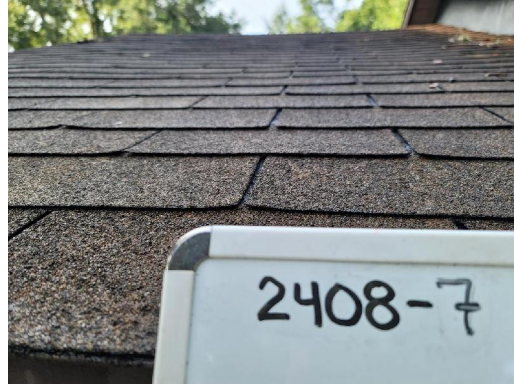
2408-7 Asphalt Shingle/Brown Typical Exterior Roof
