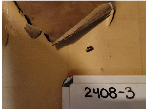
2408-3 Linoleum/Yellow Bathroom (30 sq ft)
