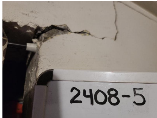
2408-5 Plaster Typical Interior Walls
