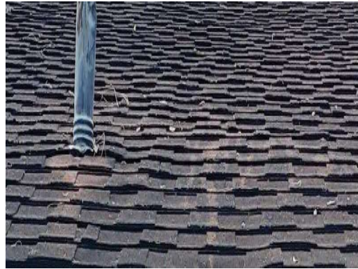
917-1 Asphalt Shingle/Mastic Typical Exterior Roof
