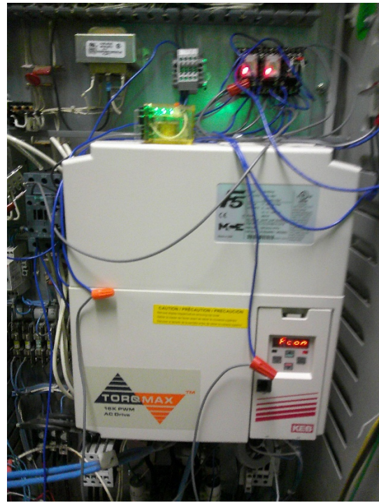
Replaced AC drive wiring that needs to be cleaned up and professional installed. This wiring is NOT acceptable.
