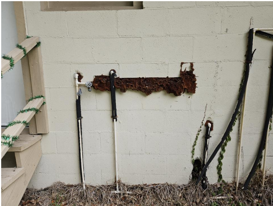
Image 2- Existing conditions - plumbing.
