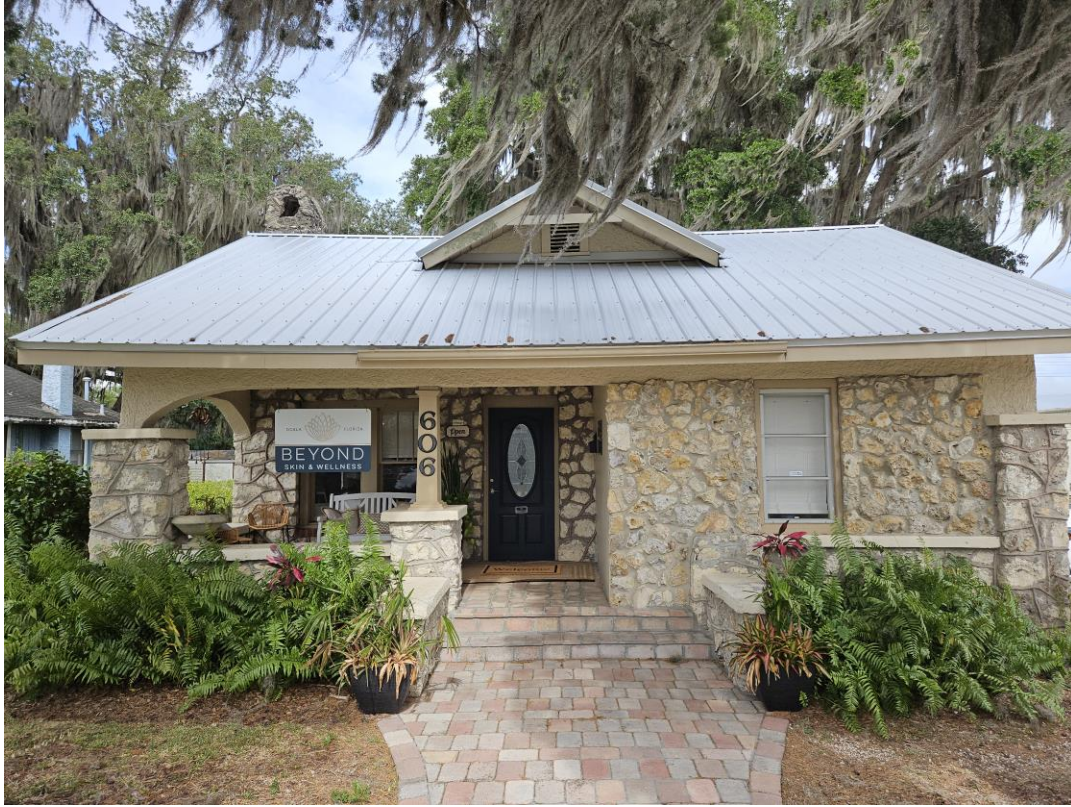
Image 1- Existing conditions- façade.
