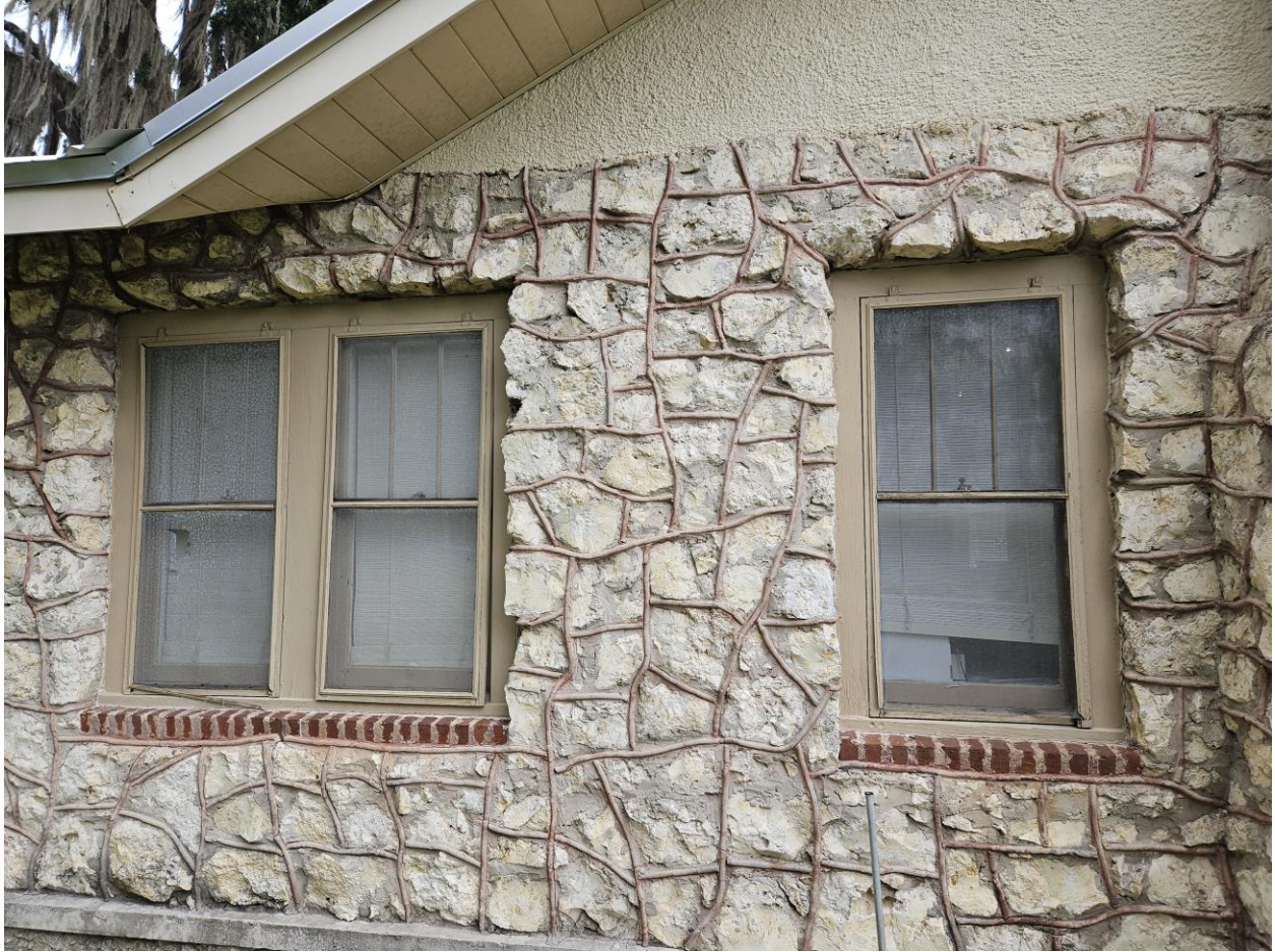
Image 2- Existing conditions – windows.
