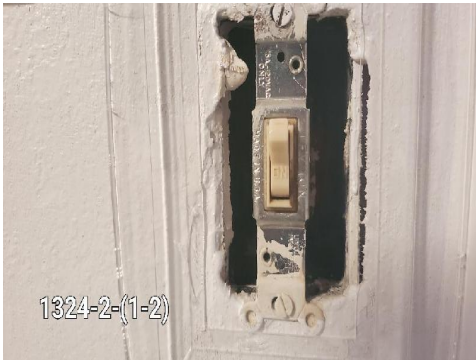
1324-2 (1-2) 1324-2 Drywall/Joint Compound/Cream Typical Interior Walls, Ceilings
