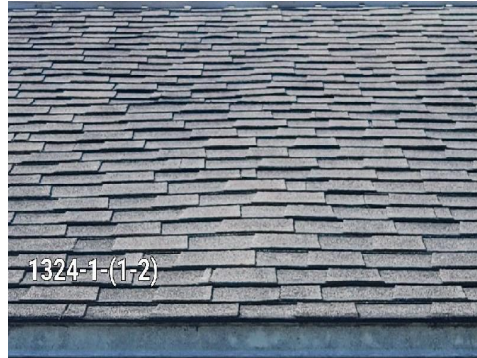
1324-1 (1-2) 1324-1 Asphalt Shingle/Gray, Tar/Black Typical Exterior Roof
