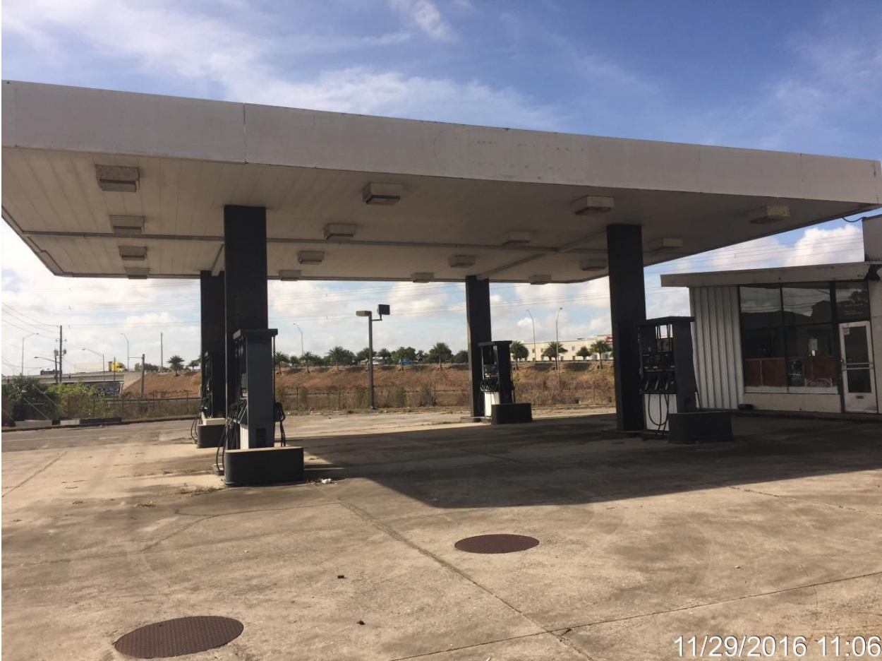
PHOTO – DEMOLISHED STRUCTURE FROM PREVIOUS USE
