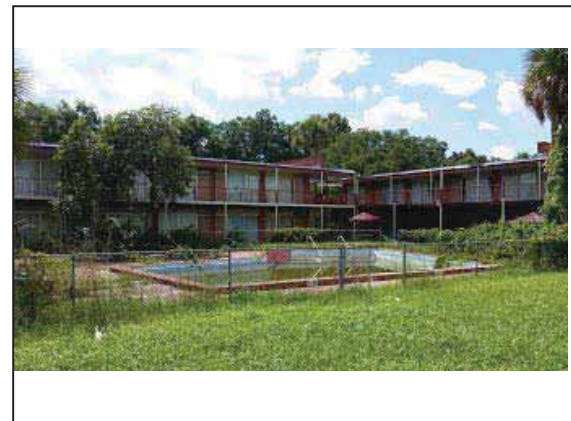
Dilapidated Motel - Ocala, FL
