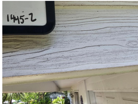
1445-2 Fibrous Siding Typical Exterior Walls
