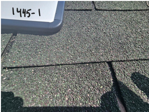
1445-1 Asphalt Shingle/Tar Typical Exterior Roof
