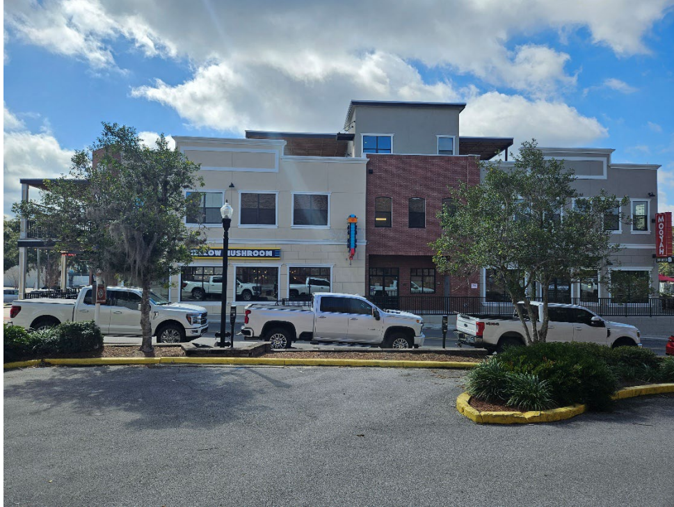
Figure 60. North elevation after completion.
