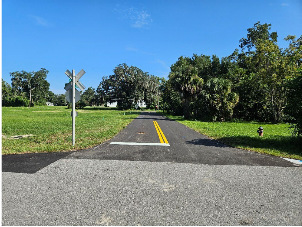
Figure 14. Newly constructed road.
