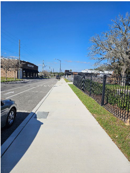
Figure 26. Sidewalk improvements along NE 1 st Avenue.
