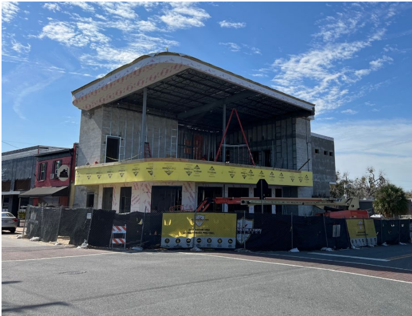
Figure 63. Construction - in progress.
