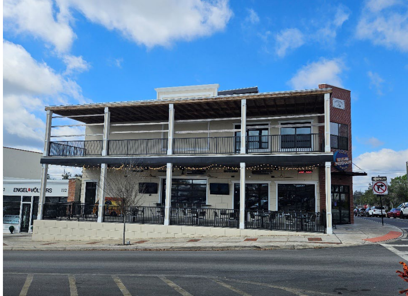
Figure 58. East elevation after completion.
