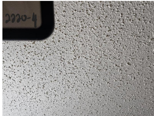
2220-4 Surfacing Texture (3% Chrysotile) Typical Interior Walls/Ceilings
