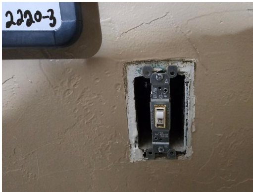
2220-3 Joint Compound (2% Chrysotile) Drywall Typical Interior Walls/Ceilings
