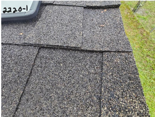
2220-1 Asphalt Shingle/Tar Typical Exterior Roof
