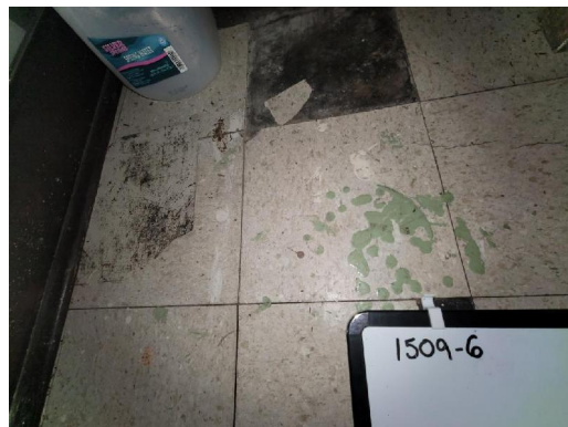
1509-6 9"x9" Floor Tile/Tan (2% Chrysotile) Mastic/Black (5% Chrysotile) Interior West Bedroom (Appx. 65 sf)
