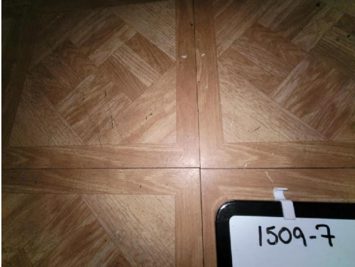
1509-7 12"x12" Floor Tile/Gray Mastic/Yellow (2% Chrysotile) Interior North Bedroom (Appx. 230 sf)
