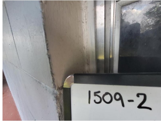
1509-2 Glazing/Tan (2% Chrysotile) Caulk Typical Exterior Windows
