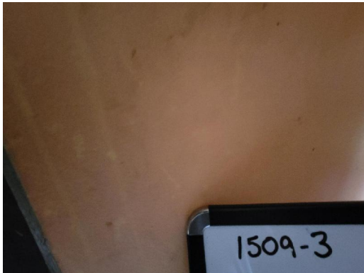
1509-3 Drywall/Joint Compound Typical Interior Walls/Ceilings
