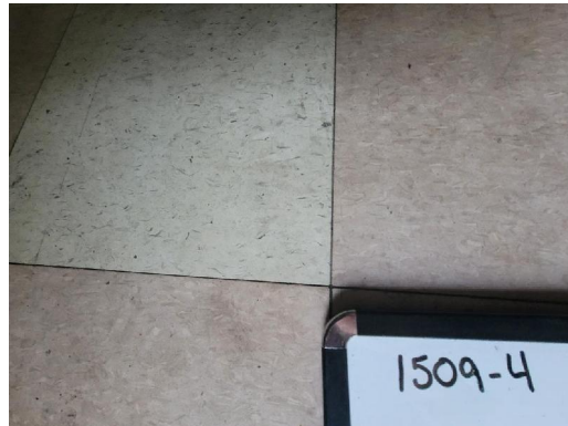
1509-4 12"x12" Floor Tile/White/Brown Mastic/Black (3% Chrysotile) Interior Living Room (Appx. 168 sf)
