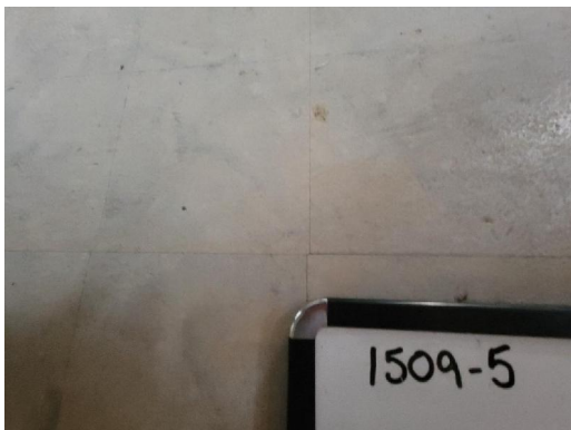
1509-5 Rolled Flooring/Mastic Interior Dining Room
