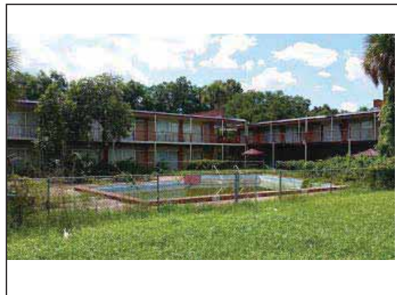
Dilapidated Motel - Ocala, FL
