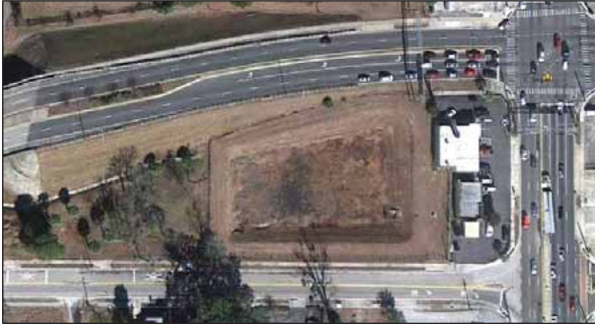
SR40 and Pine Ave DRA before reduction and relocation to provide for redevelopment of catalytic site.
