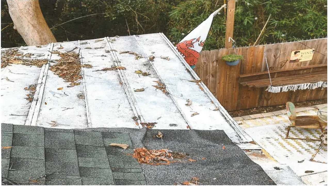
Image 2 -Existing condition - metal section.
