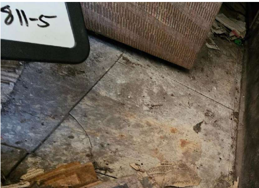
811-5 12"x12" Floor Tile Typical Interior
