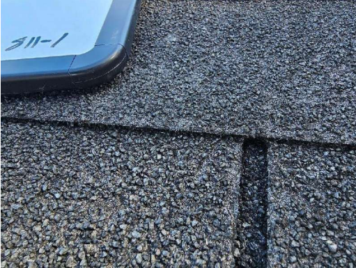
811-1 Asphalt Shingle/Tar Typical Exterior Roof
