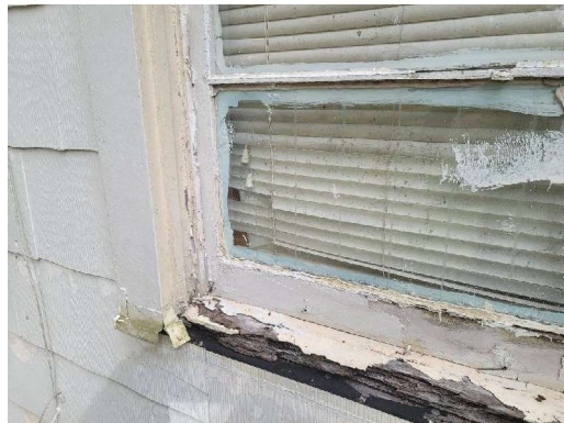
Exterior(009) D-Wall, Right Wood Window Components Lead-Positive, Deteriorated
