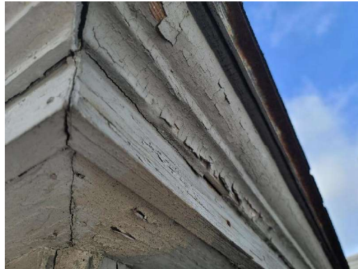
Exterior(009) C-Wall, Center Wood Soffit and Fascia Lead-Positive, Deteriorated
