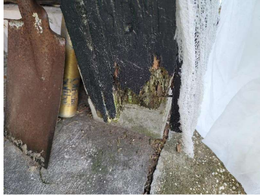
Exterior(009) A-Wall, Left Wood Garage Door Jamb Lead-Positive, Deteriorated
