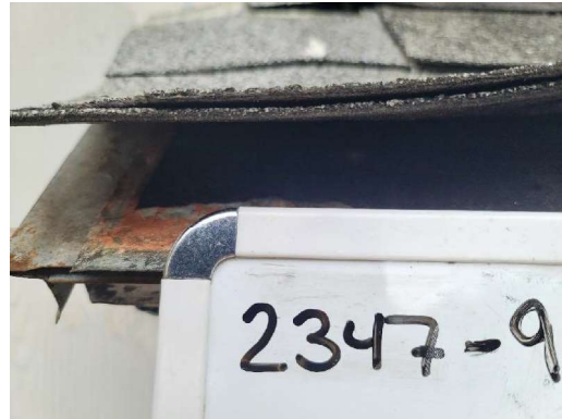
2347-9 Rolled Roofing Typical Exterior Roof
