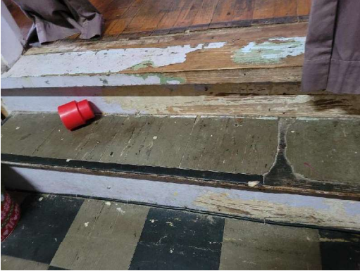
Bedroom A(002) D-Wall, Right Wood Stair Tread and Riser Lead-Positive, Deteriorated
