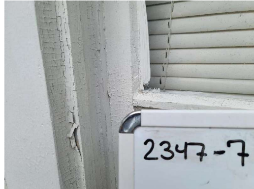
2347-7 Window Glazing (<1% Chrysotile) 5 Exterior Windows
