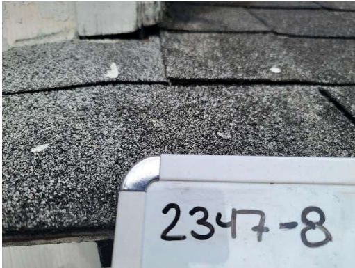
2347-8 Asphalt Shingle Typical Exterior Roof
