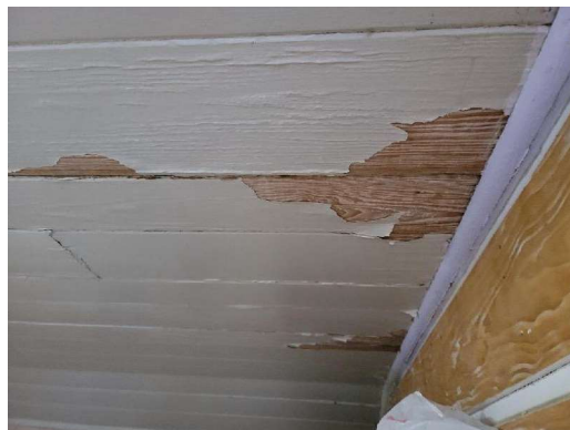
Bedroom A(002) D-Wall, Center Wood Ceiling Lead-Positive, Deteriorated
