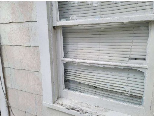
Exterior(009) C-Wall, Left Wood Window Components Lead-Positive, Deteriorated
