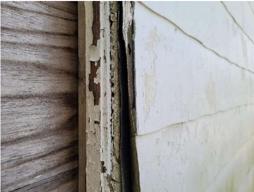
Exterior(009) B-Wall, Left Wood Door Jamb Lead-Positive, Deteriorated
