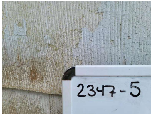
2347-5 Transite Siding (10% Chrysotile) Typical Exterior Walls
