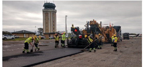
Taxiway "A" Construction
