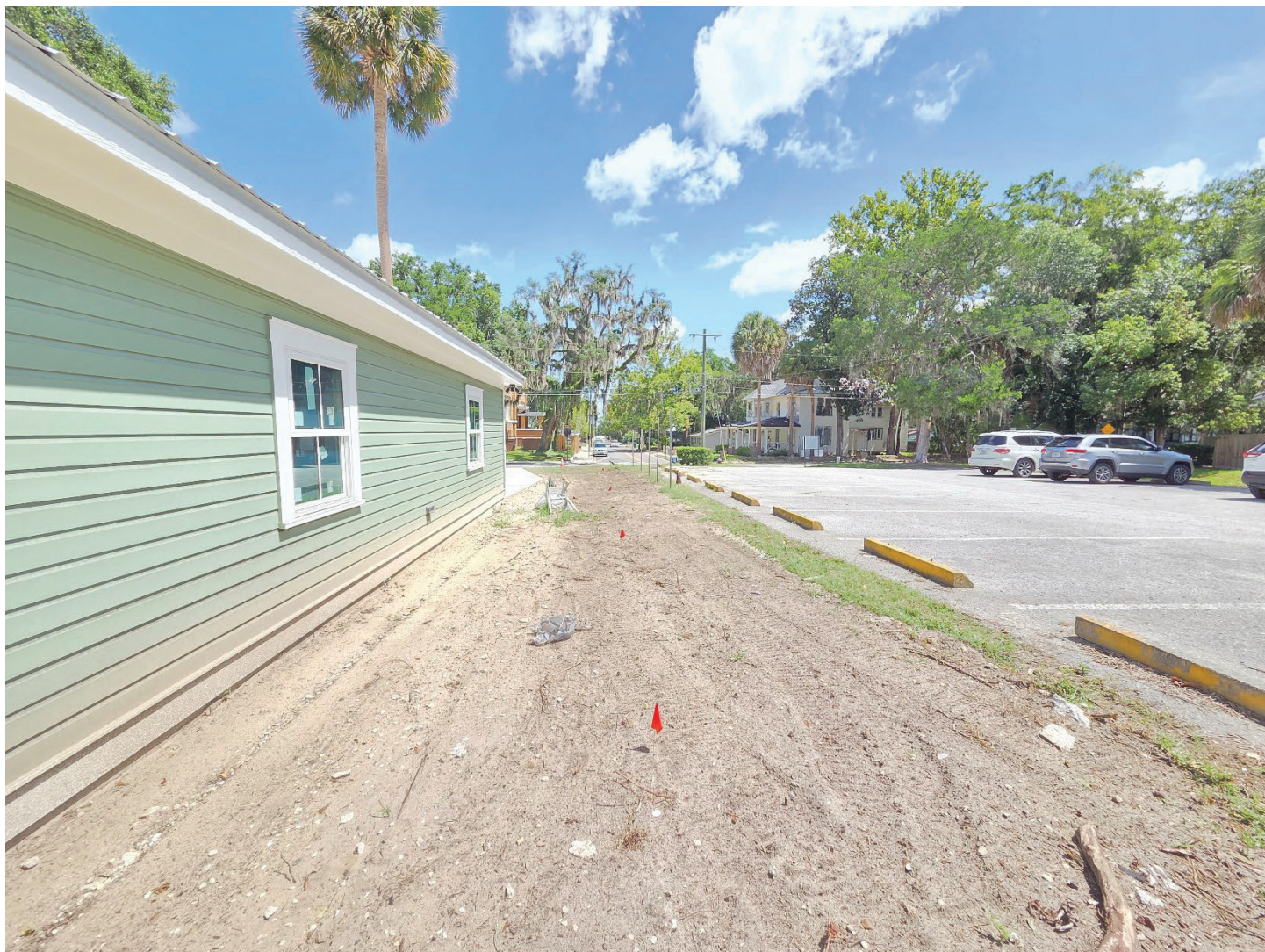
The eastern property line of the property where a section of the fence will be installed facing north
