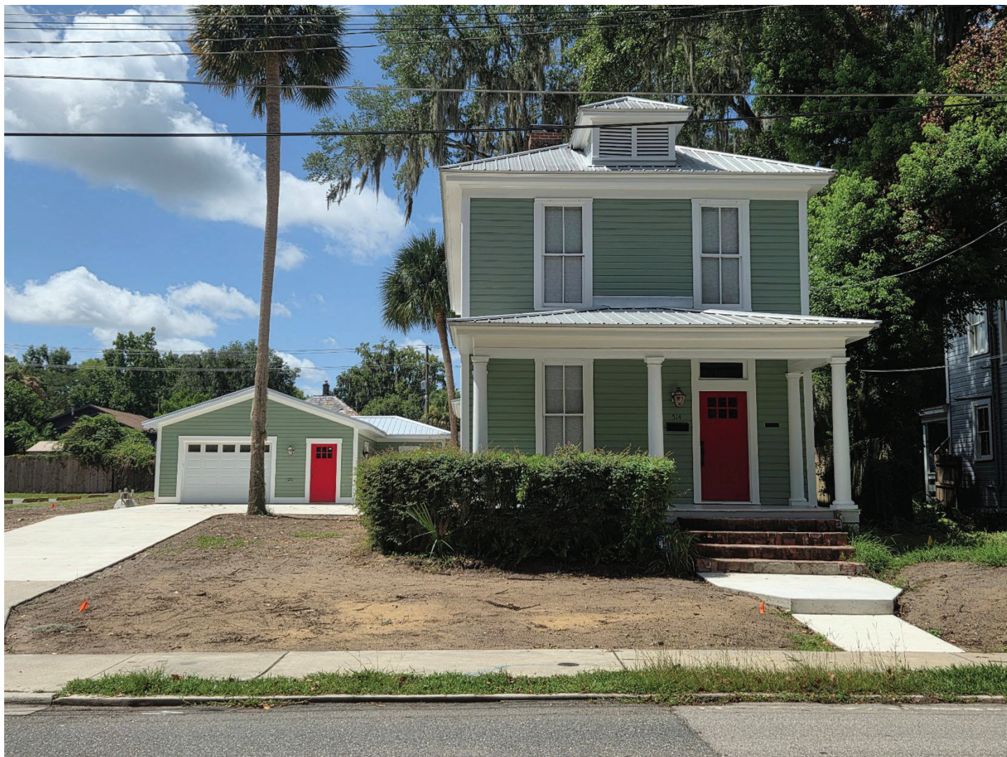
514 SE 8 th Street from SE 8 th Street facing south
