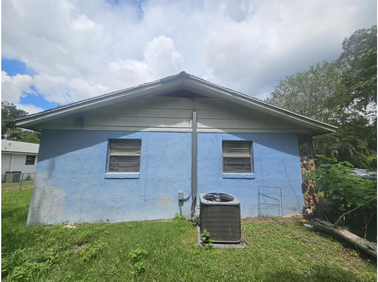
Image 3- View of the back of the home
