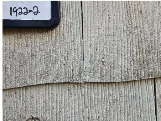
1922-2 Transite Siding/Gray (13% Chrysotile) Typical Exterior Walls
