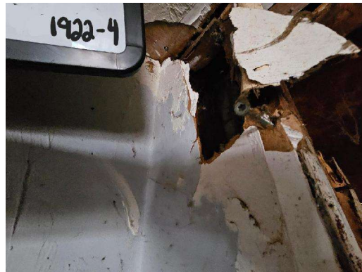
1922-4 Drywall/Joint Compound Typical Interior Walls/Ceilings
