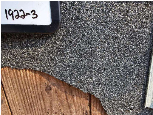
1922-3 Asphalt House Wrap Typical Exterior Walls
