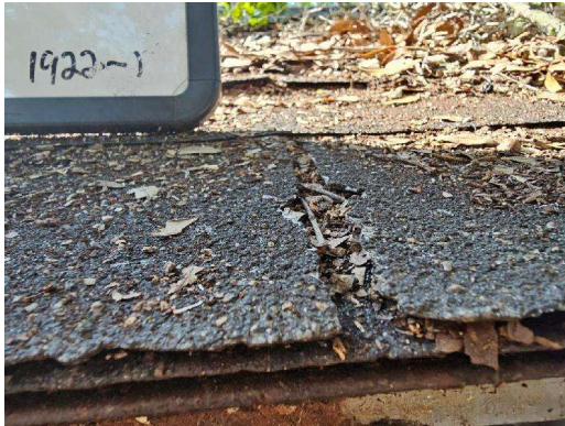
1922-1 Asphalt Shingle Typical Exterior Roof
