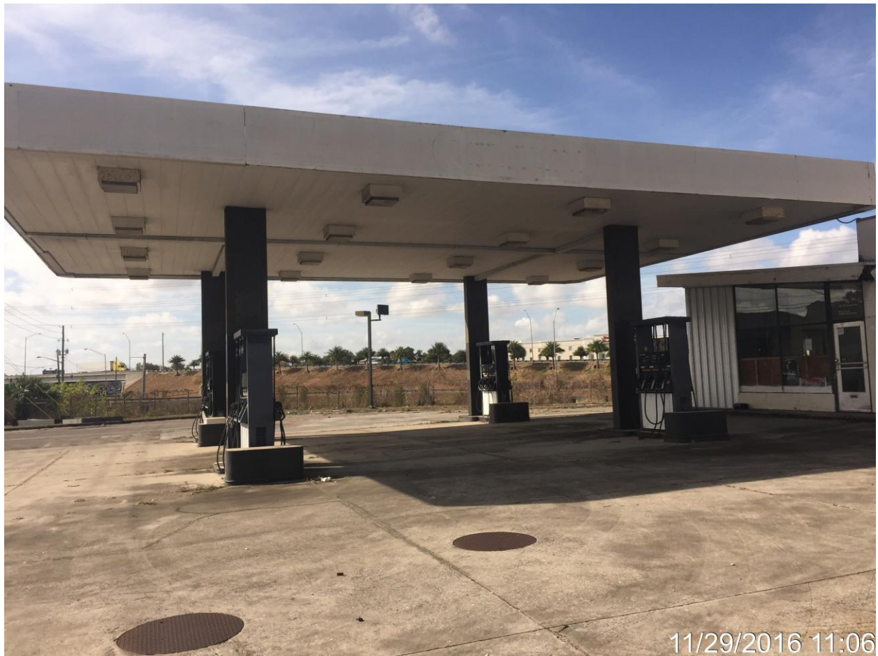
PHOTO – DEMOLISHED STRUCTURE FROM PREVIOUS USE
