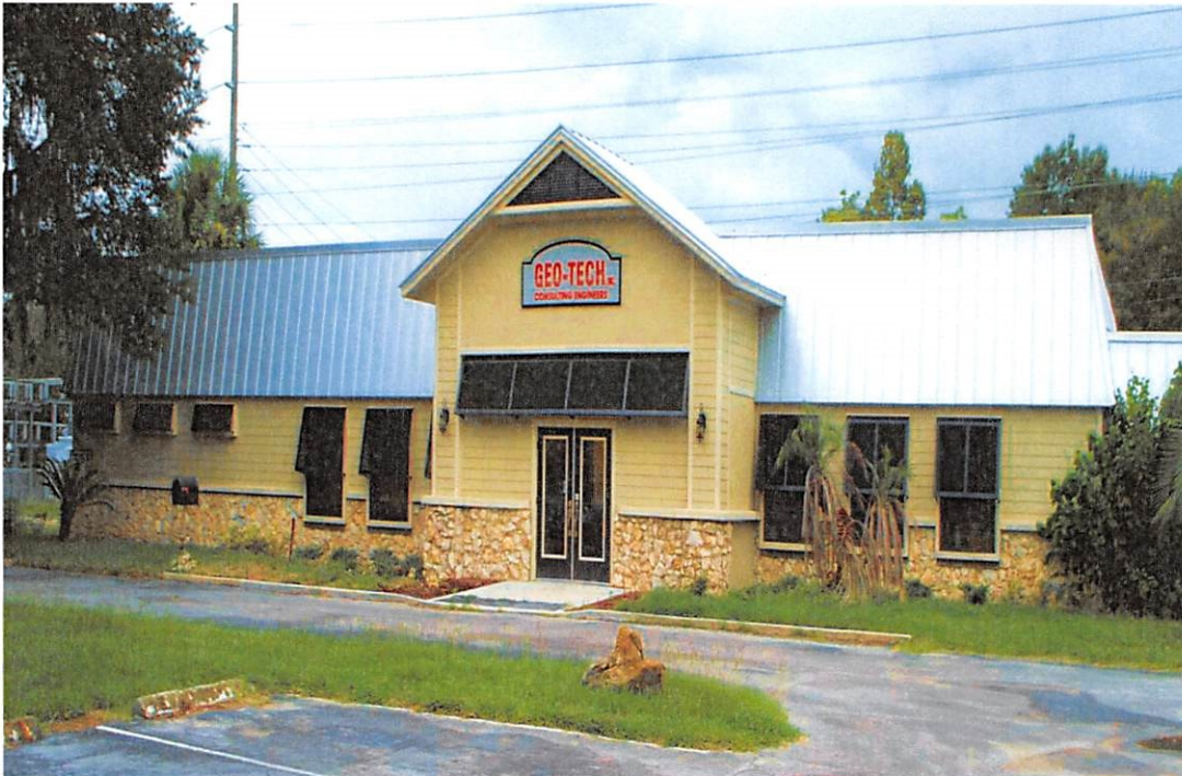
Geo-Tech's Corporate Office: 1016 SE 3 rd Avenue in Ocala, Florida Phone: 352-694-7711 FID No.: 59-3576170
