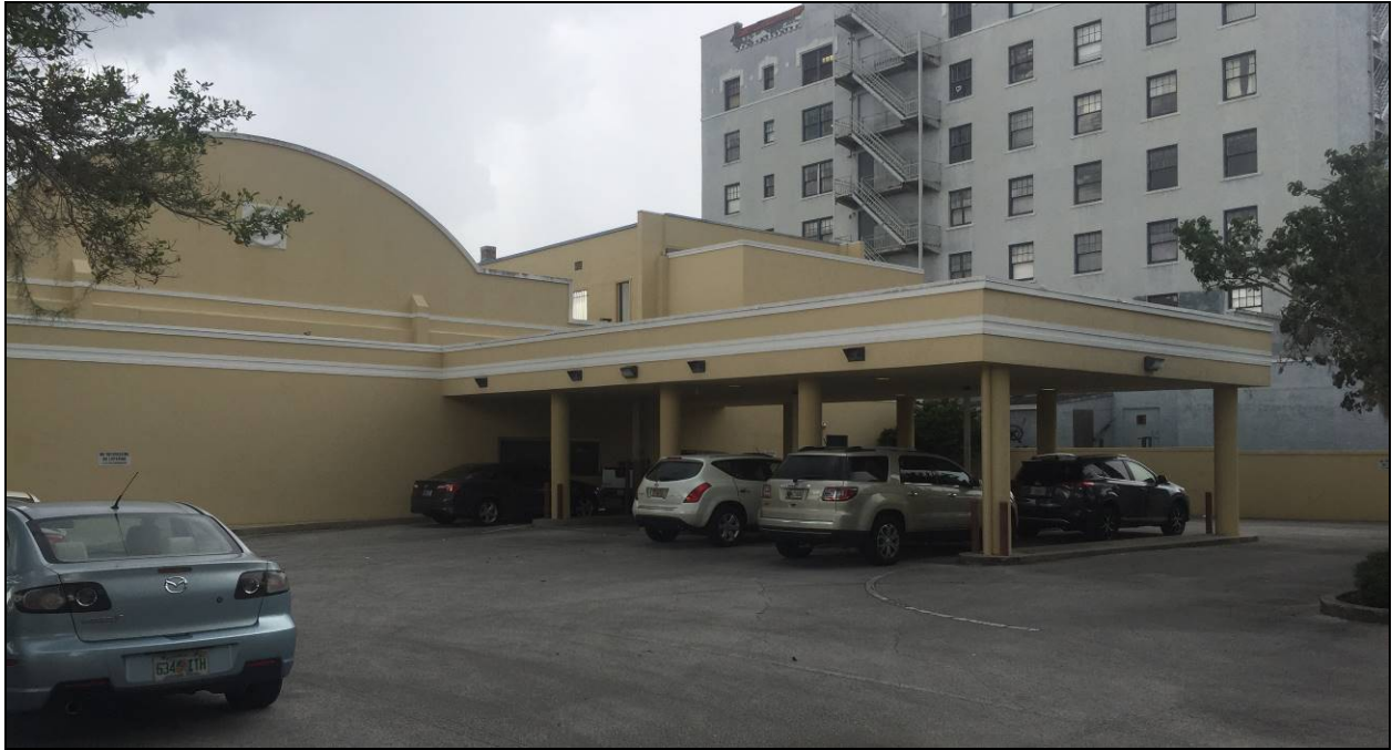
The drive-thru canopy was added in 1997, comprises (4) lanes, and is used for employee parking.
