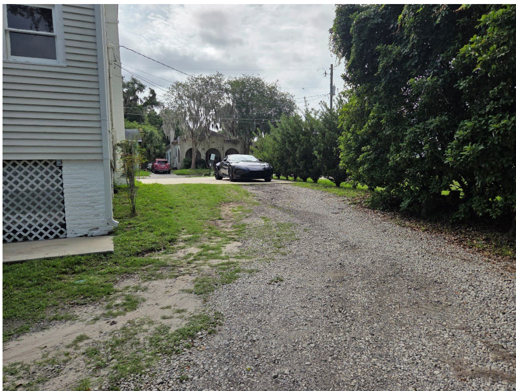
Existing concrete pad and driveway on the west side of the property
