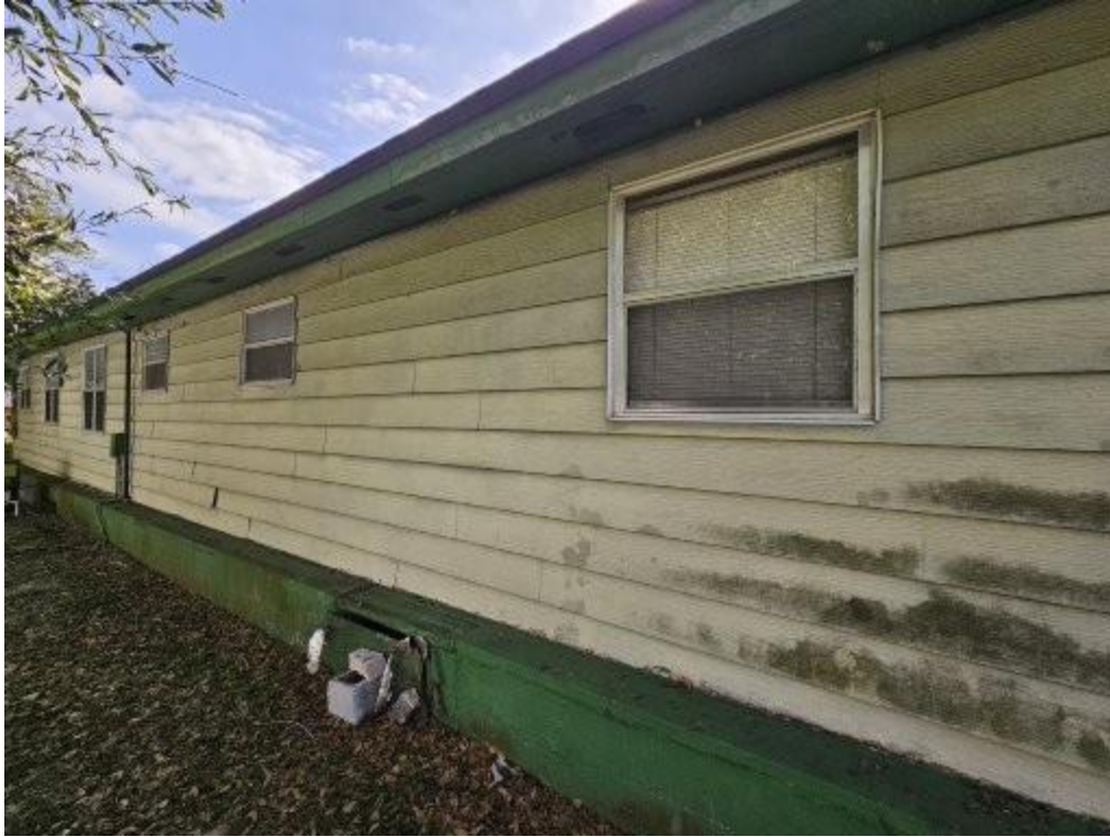
Image 3 – Existing conditions of windows and building façade.
